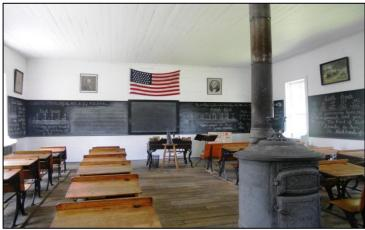
The interior walls and ceiling are wood and in good condition. The floor is wood board and although it looks rough, is also in good condition. Interior doors have been replaced with new wood doors and they are in good condition. The architectural woodwork around the windows is in good condition.
