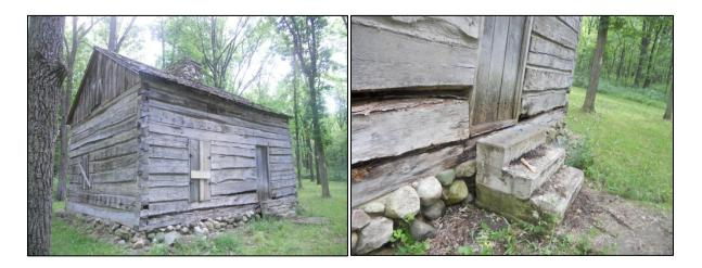
The roof is wood shake with organic plant material taking root. The plant material should be removed to protect the wood. The chimney is rubble stone to match the foundation and appears to be in good condition.
