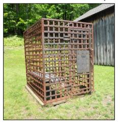
The wooden bench inside the cell is split and in poor condition due to its exposure to the elements. This is more easily replaced as needed than the elegant metal framework. Since it is unpainted and should remain unpainted, it would not be advisable to replace it with plastic material or fiber cement board.
