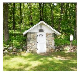
The spring house is constructed of stone with mortar joints and is built into the side of the hill. There is painted wood board and batten siding with a vent and a plaque about the door in the gable. The door is wood and is new. The roof is asphalt shingle. Overall, this building is in excellent condition and should require minimal maintenance within the next 10+ years.
