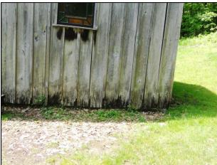
Some of the battens have pulled away, granting animals access to the building's interior. These should be replaced with new battens to match existing. There are some wood framed stained glass windows located in the building that are not original, but are in good condition. Two large, new double entry doors allow public access to the display and demonstration space. The roof is asphalt shingle and in excellent condition. It appears to be quite new.
