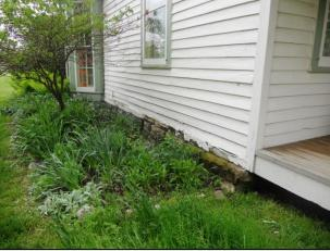
When the source of the issue is resolved, the stone should be lightly cleaned with a scrub brush, water, and detergent. The skirt board could be replaced with a milled to shape, paintable fiber cement board or recycled plastic board so that further maintenance is reduced. Any damage to the structural member below should be repaired.
