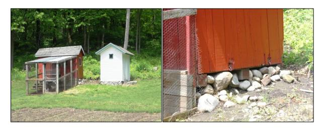
The siding is vertical wood siding in okay to good condition. It's painted and fairly well maintained. The wood door and windows into the coop area are in okay to good condition. The side windows have chicken wire over them for further ventilation if desired. The wood shingles over the coop are okay to good condition. This roosting area appears to stay dry.
