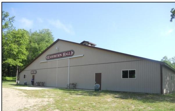
This is a pole barn built on a concrete slab on grade with treated lumber. The exterior walls are plywood/particle board with vinyl panel siding on the exterior. The wood structure is exposed on the interior of the building. Doors are wood and metal. Windows are aluminum. The roof is asphalt shingle and the wood underlaying is dry. All appear to be in excellent condition.
