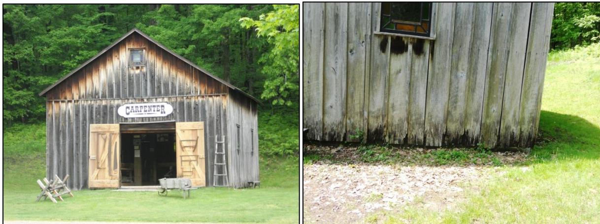
Some of the battens have pulled away, granting animals access to the building's interior. These should be replaced with new battens to match existing. There are some wood framed stained glass windows located in the building that are not original, but are in good condition. Two large, new double entry doors allow public access to the display and demonstration space. The roof is asphalt shingle and in excellent condition. It appears to be quite new.
