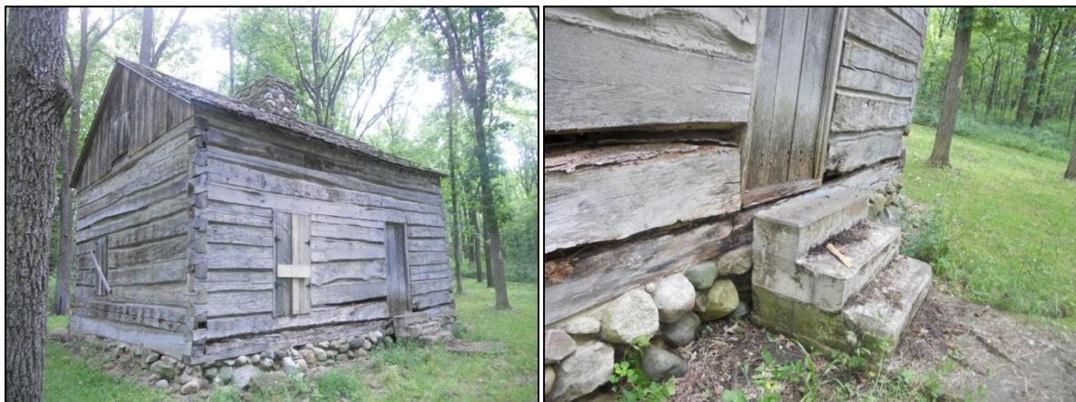
The roof is wood shake with organic plant material taking root. The plant material should be removed to protect the wood. The chimney is rubble stone to match the foundation and appears to be in good condition.
