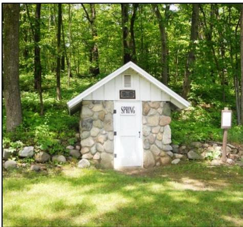
The spring house is constructed of stone with mortar joints and is built into the side of the hill. There is painted wood board and batten siding with a vent and a plaque about the door in the gable. The door is wood and is new. The roof is asphalt shingle. Overall, this building is in excellent condition and should require minimal maintenance within the next 10+ years.
