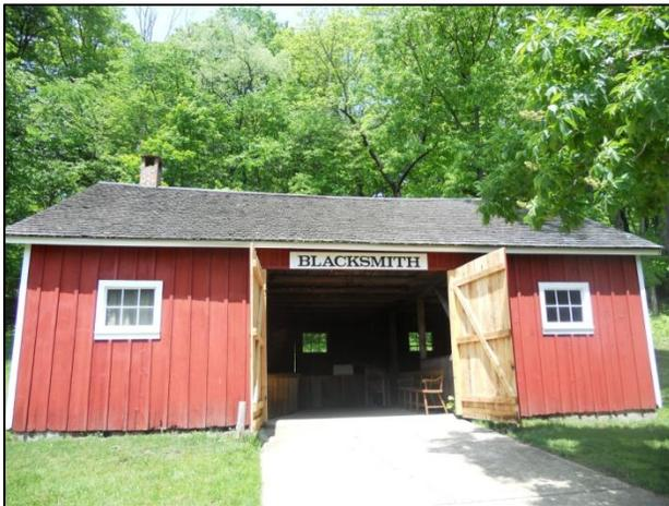
There are a number of wood framed, multi-paned glass windows located in the building that are in good condition. Two large, new double entry doors allow public access to the display and demonstration space. The roof is wood shake and in fair to good condition. A long term plan for this building should include a plan to replace the roof. If it is not feasible to replace the wood shakes with new wood shakes, it is recommended that a metal roof be installed in its place.
