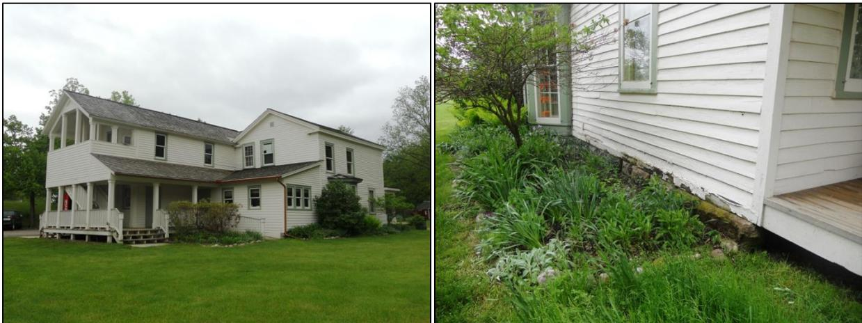
When the source of the issue is resolved, the stone should be lightly cleaned with a scrub brush, water, and detergent. The skirt board could be replaced with a milled to shape, paintable fiber cement board or recycled plastic board so that further maintenance is reduced. Any damage to the structural member below should be repaired.
